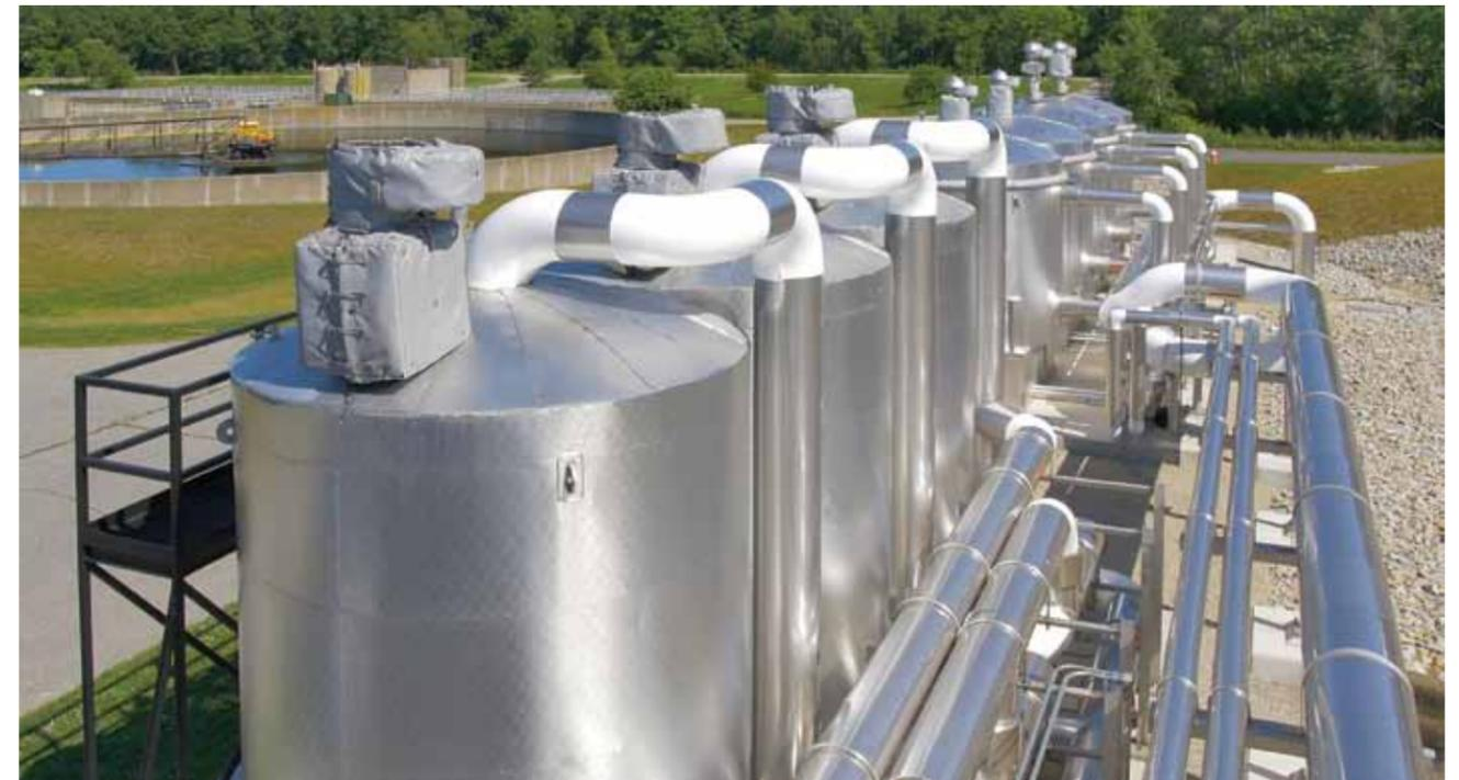
Biogas is treated for H<sub>2</sub>S and siloxane removal prior to beneficial use
